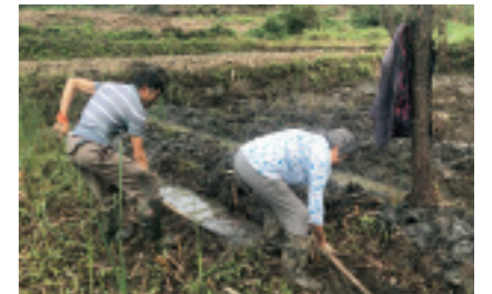
Community participation in the construction of "S-bend" wetland
