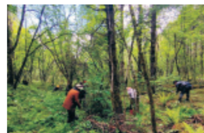
Forest and Brush Clearing in Xiaoxiangling Mountains project site
