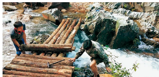
■ Patrolmen are repairing bridges
